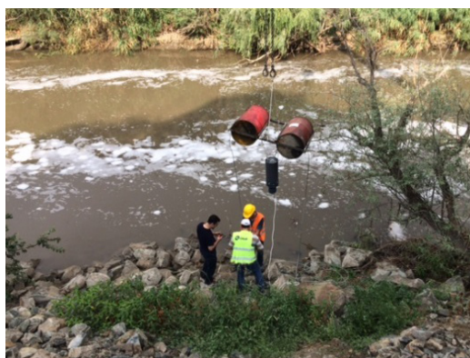
Application of MICRA in a hydropower project
